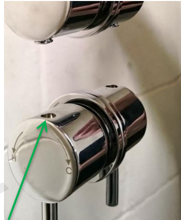
1. Remove the Temperature Handle concealing cap.
