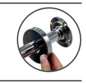
nsuring the rubber washer is in the correct position, attach the shower head to the fixed arm and carefully secure using a suitable spanner, or a tool with smooth jaws, sufficiently to lock the head into position.
