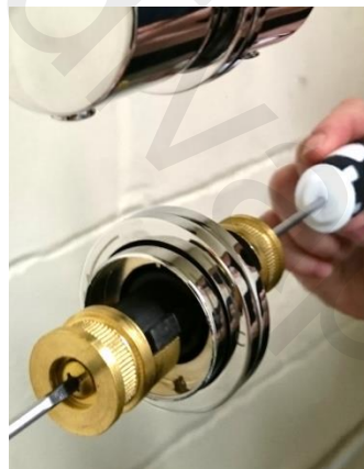
4. Using a Cross-head screwdriver remove the Handle Bush.
