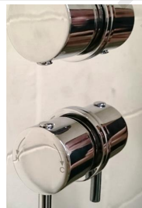
9. Re-fit the Temperature Handle Concealing cap.
