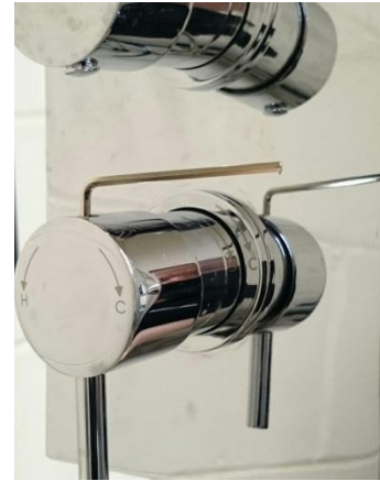
2. Using the 2.5mm Allen key provided loosen the grub screw and remove the Temperature Handle.*
