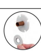
Trim the projecting pipe to a length of 15-22mm, measured from the face of the gripper ring, using a suitable cutter. If a hacksaw is used, the pipe end must be carefully de-burred and chamfered.
