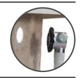
insuring the rubber washer is correctly aligned, pass the overflow filler outlet through the bath and secure to the body assembly.
