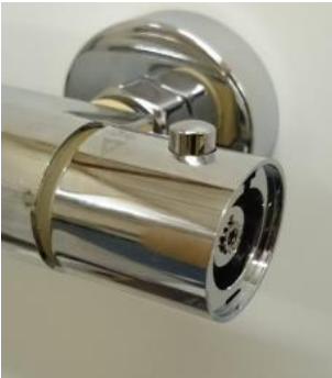
4. Relocate the Temperature Handle back onto the Cartridge Spline by approx. 3mm.
