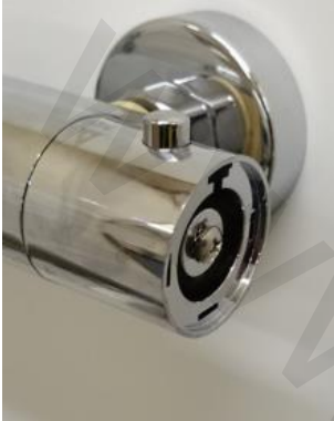
1. Remove the Temperature Handle Concealing Cap.
